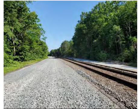
Location: Hoosick, NY Owner: Pan Am Southern Completion: Ongoing
