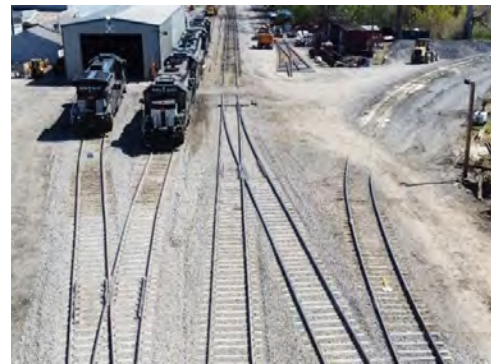
Location: Waterloo, NY Owner: Finger Lakes Railway Completion: 2021
