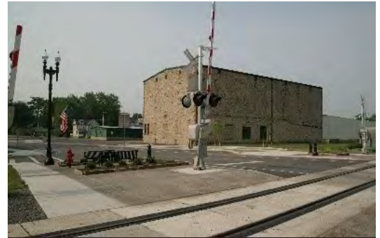
Location: Medina, NY Owner: Falls Road Railroad
