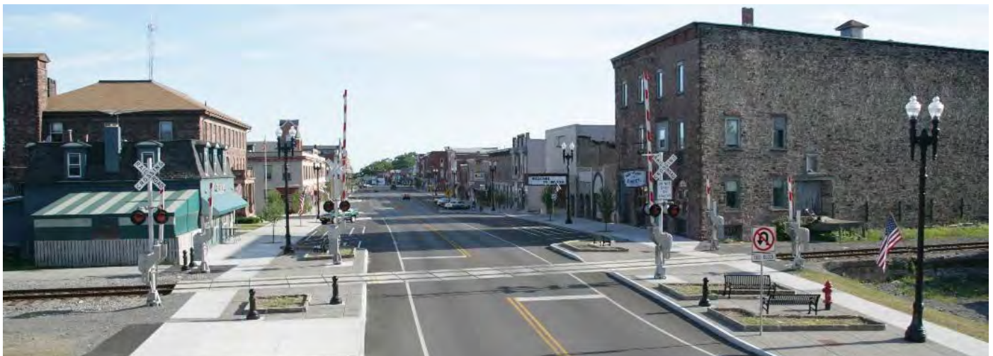
Grade crossing surface, signal, and curb delineation improvements were provided at the Main Street crossing.
