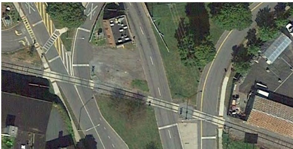
Aerial overview of three successive grade crossings at the interchange.
