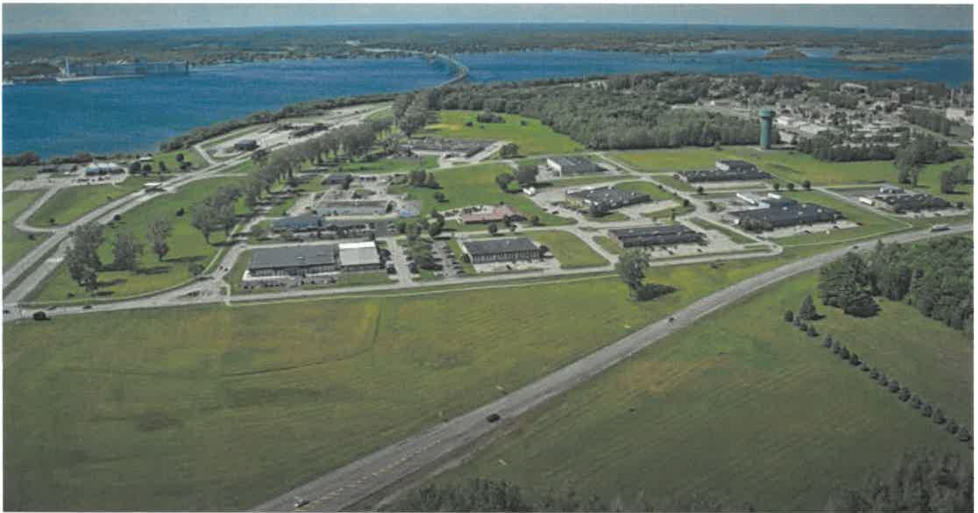
The Ogdensburg Bridge and Port Authority Commerce Park on Route 37. Christopher Lenney/Watertown Daily Times
