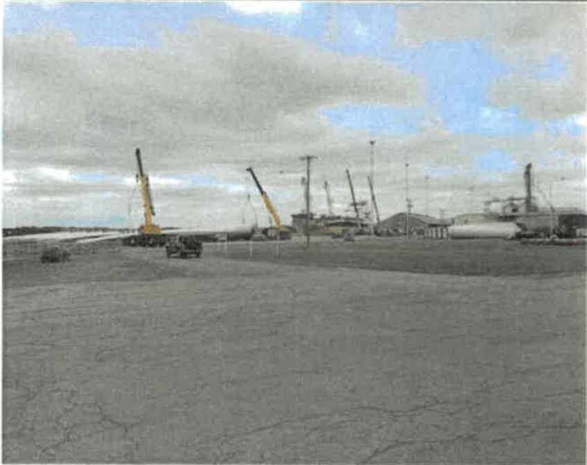
9 Cranes in use- 7 Shore Cranes/ 2 Vessel cranes
