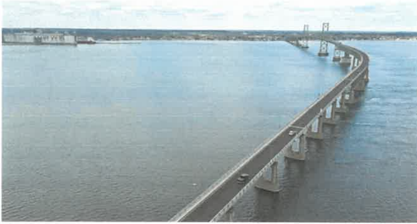
Sparse traffic crosses the Ogdensburg-Prescott International Bridge. Christopher Lenney/Watertown Daily Times
