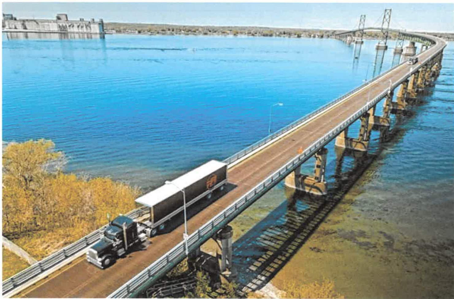
The Ogdensburg-Prescott International Bridge. Christopher Lenney/Watertown Daily Times
