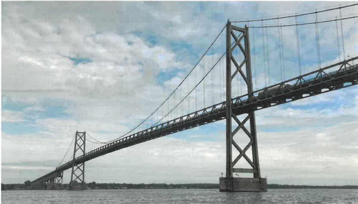
FIGURE 1: Parsons successfully delivered the previous set of 2020-2023 biennial and special inspections and load ratings for the OBPA and we are well prepared to do it again.
